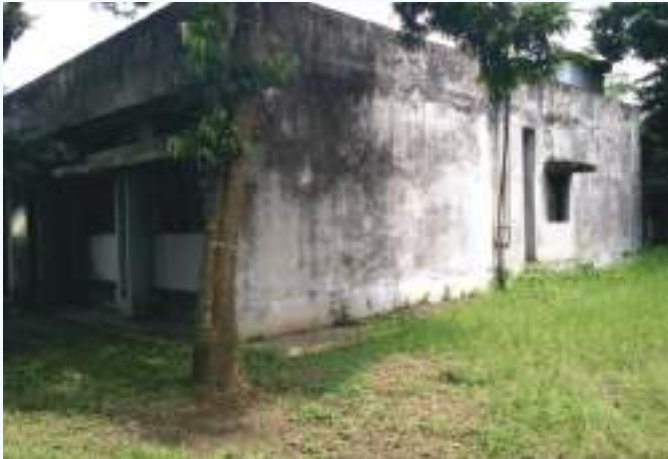
Outside view of the RFTL
