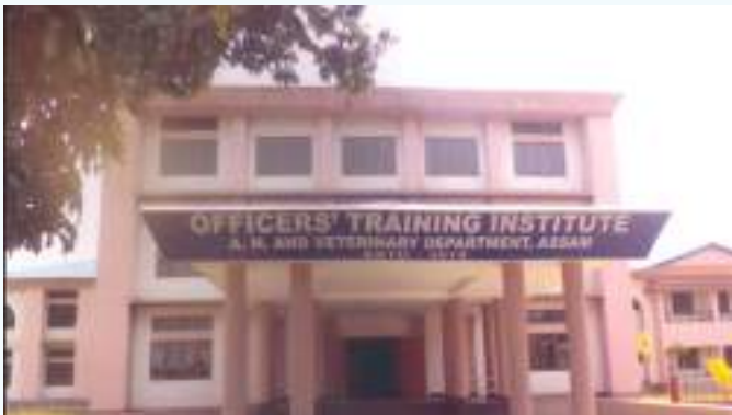
Main Building, OTI, Khanapara
