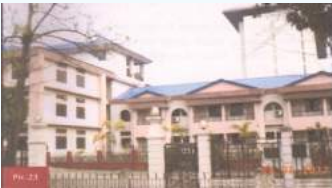
Main Building, OTI, Khanapara
