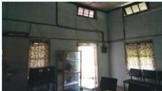
School Building, Ghungur
