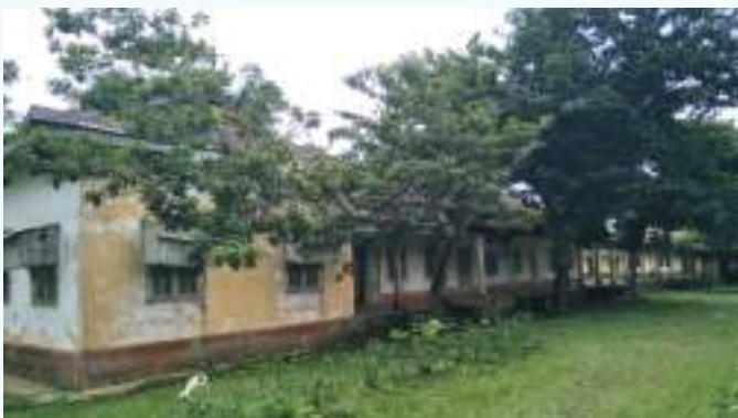
School Building, Ghungur
