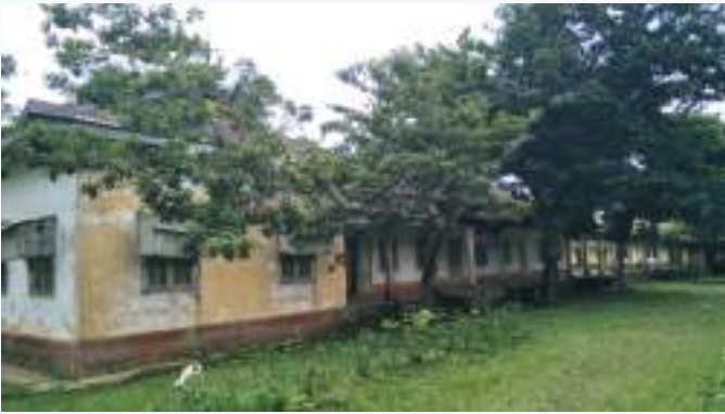
School Building, Ghungur
