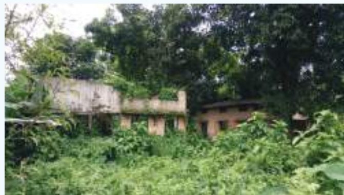
Damaged buildings, Veterinary Training centre at Demow
