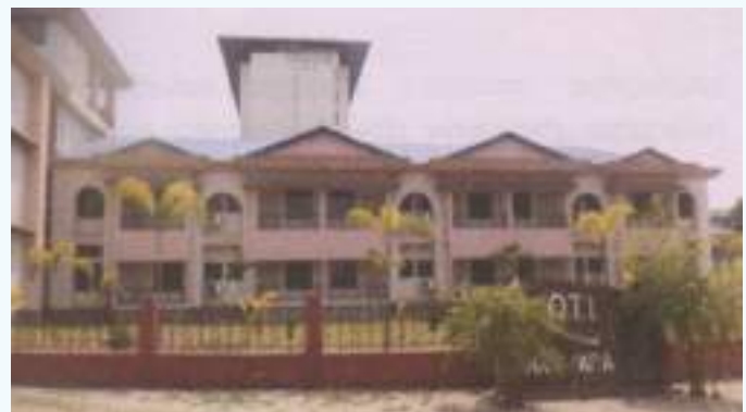
Main Building, OTI, Khanapara
